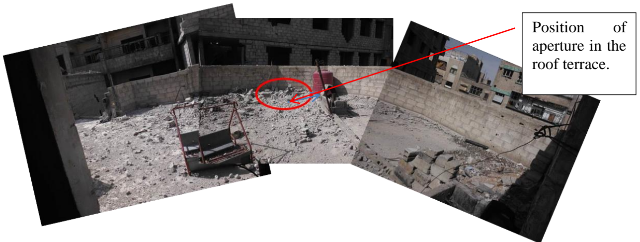
FIGURE A.7.3 ROOF OF LOCATION 4
